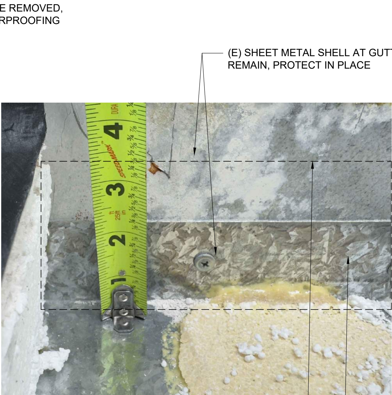
NOTE: 1. ALL (E) EXPOSED FASTENERS TO BE REMOVED AND REPLACED, REFER TO WP1.01 & WP1.02 EXISTING CONDITION PHOTO REFERENCE 8 WP9.02 N.T.S. DO NOT SCALE PHOTO REFERENCES.
