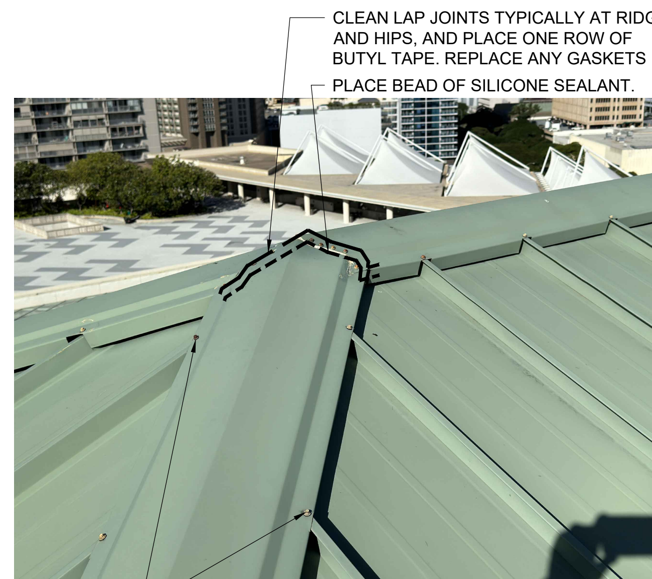
NOTE: 1. ALL (E) EXPOSED FASTENERS TO BE REMOVED AND REPLACED, REFER TO WP1.01 & WP1.02 EXISTING CONDITION PHOTO REFERENCE 11 N.T.S. DO NOT SCALE PHOTO REFERENCES. WP9.01
