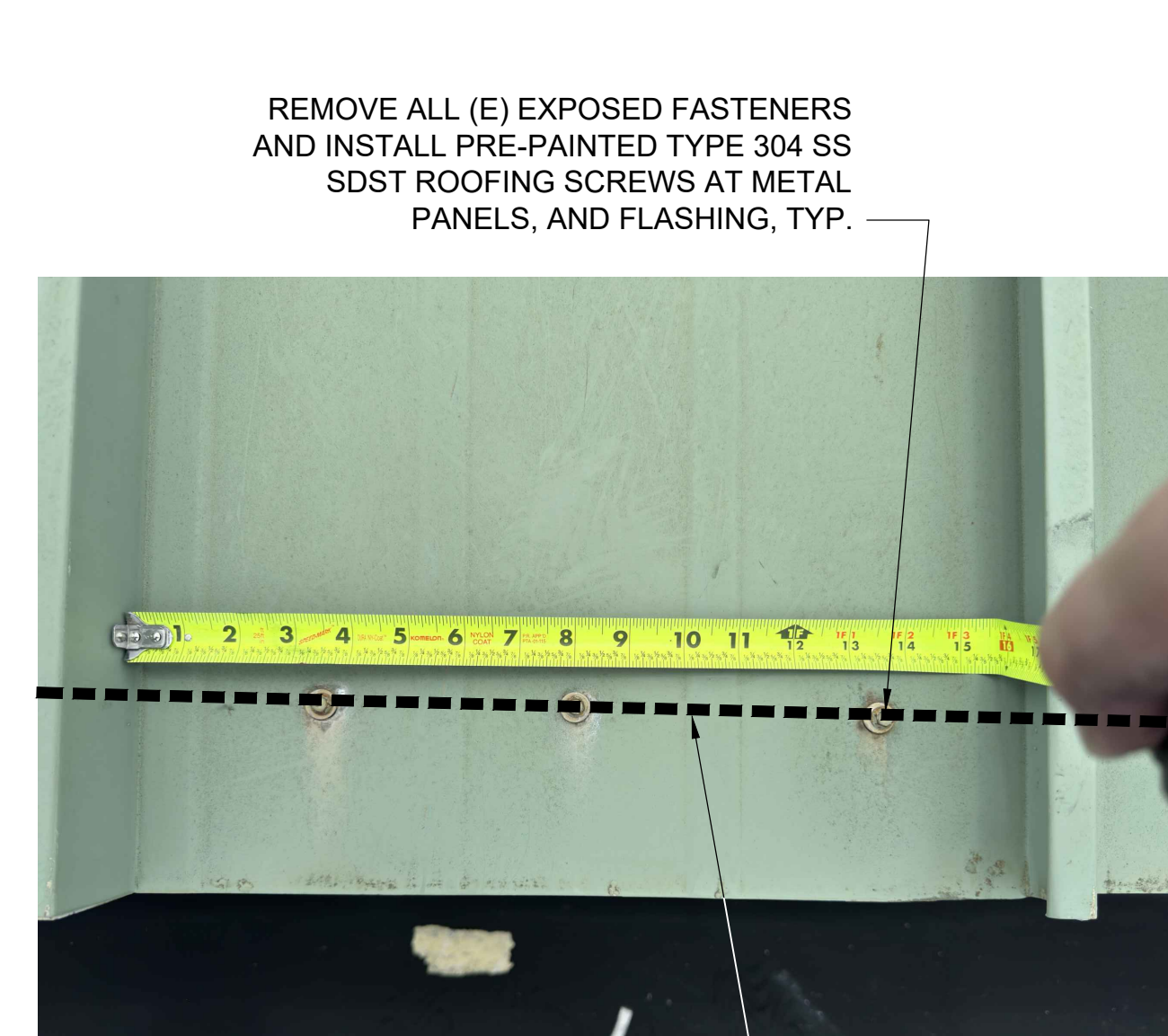
NOTE: 1. ALL (E) EXPOSED FASTENERS TO BE REMOVED AND REPLACED, REFER TO WP1.01 & WP1.02 EXISTING CONDITION PHOTO REFERENCE 2 N.T.S. DO NOT SCALE PHOTO REFERENCES. WP9.01
