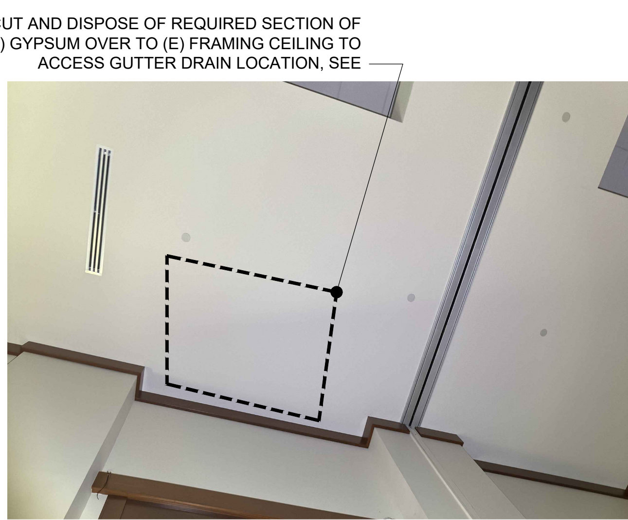
NOTES: 1. WALL MATERIALS REMOVED TO ACCESS DRAINS AND STORM DRAIN PIPING SHALL BE REPLACED WITH SAME MATERIALS IN MATCHING THICKNESS AND TYPE, AND INCLUDING TAPING AND MUDDING SEAMS TO MATCH EXISTING FINISH AND PRIMING AND PAINTING IN MATCHING COLOR. 2. REPLACE DAMAGED FIREPROOFING IN LIKE KIND. 3. SEE DETAIL 1/WP5.02 DRAIN LOCATIONS PHOTO REFERENCE 3 WP9.03 N.T.S. DO NOT SCALE PHOTO REFERENCES.
