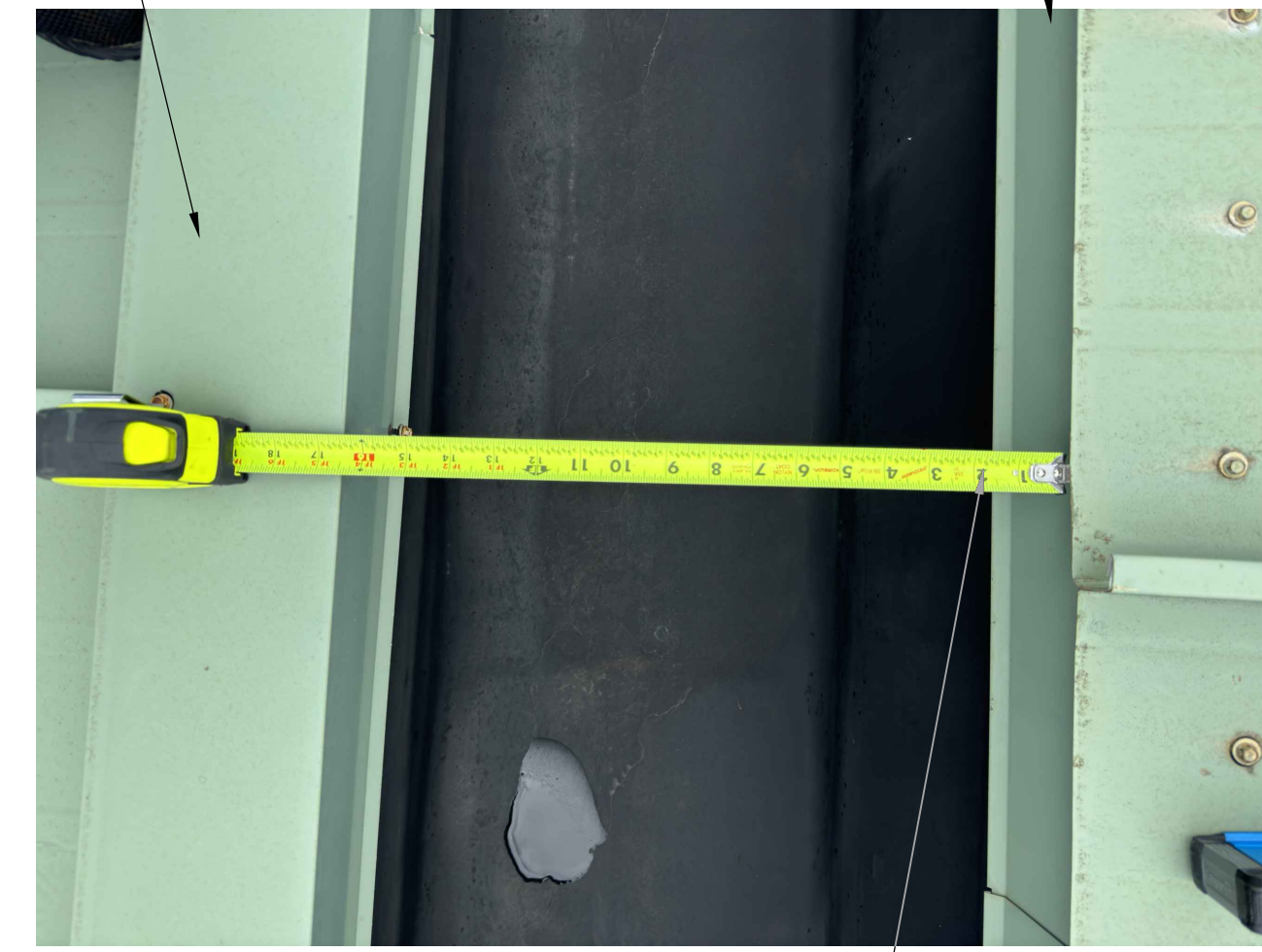
NOTE: 1. ALL (E) EXPOSED FASTENERS TO BE REMOVED AND REPLACED, REFER TO WP1.01 & WP1.02 EXISTING CONDITION PHOTO REFERENCE 4 N.T.S. DO NOT SCALE PHOTO REFERENCES. WP9.01
