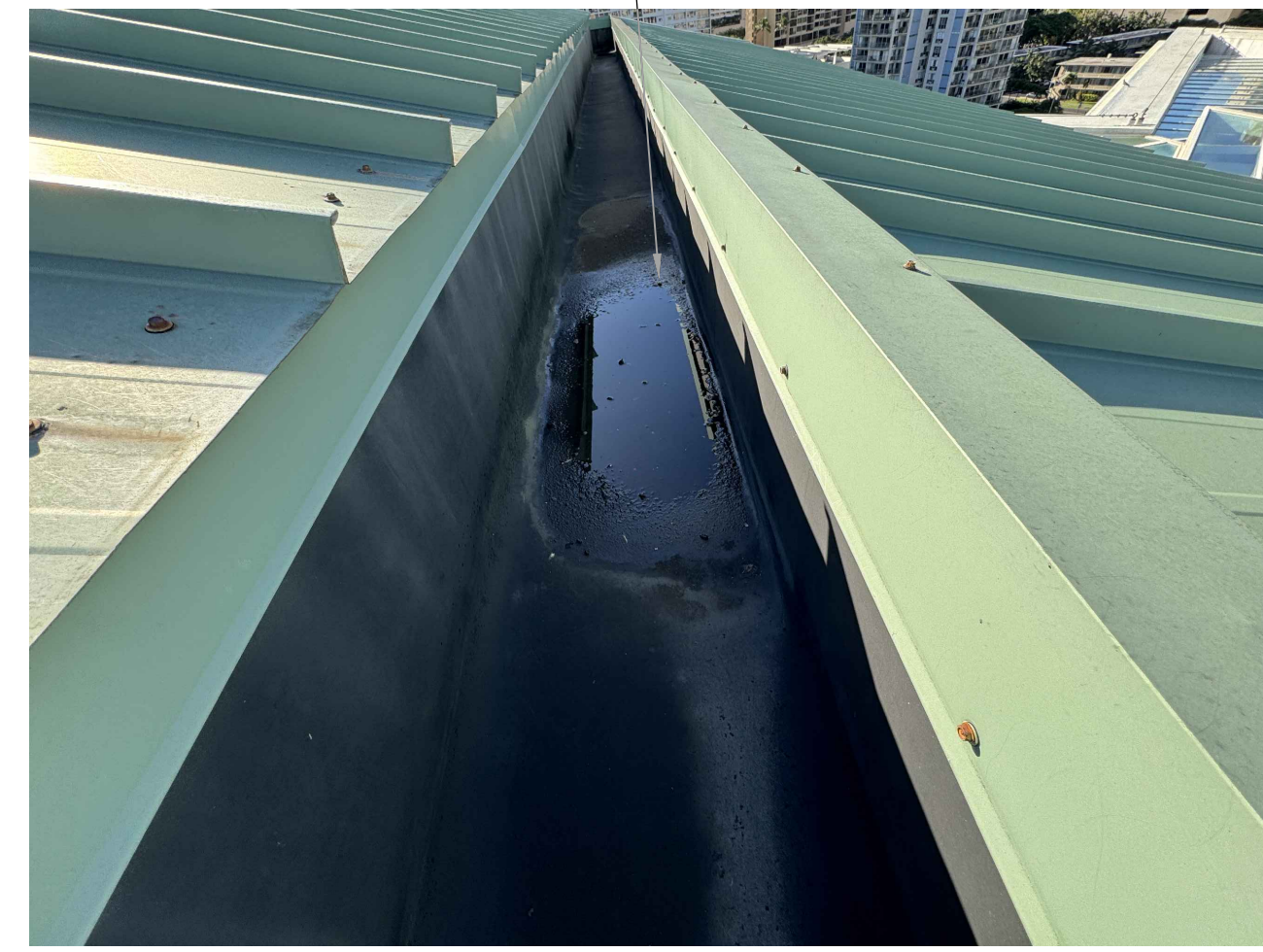
NOTE: 1. ALL (E) EXPOSED FASTENERS TO BE REMOVED AND REPLACED, REFER TO WP1.01 & WP1.02 EXISTING CONDITION PHOTO REFERENCE 10 N.T.S. DO NOT SCALE PHOTO REFERENCES. WP9.01
