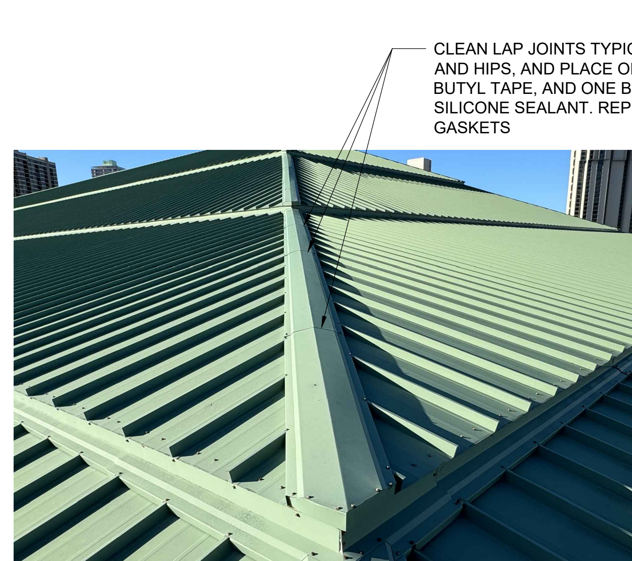
NOTE: 1. ALL (E) EXPOSED FASTENERS TO BE REMOVED AND REPLACED, REFER TO WP1.01 & WP1.02 EXISTING CONDITION PHOTO REFERENCE 11 N.T.S. DO NOT SCALE PHOTO REFERENCES. WP9.01
