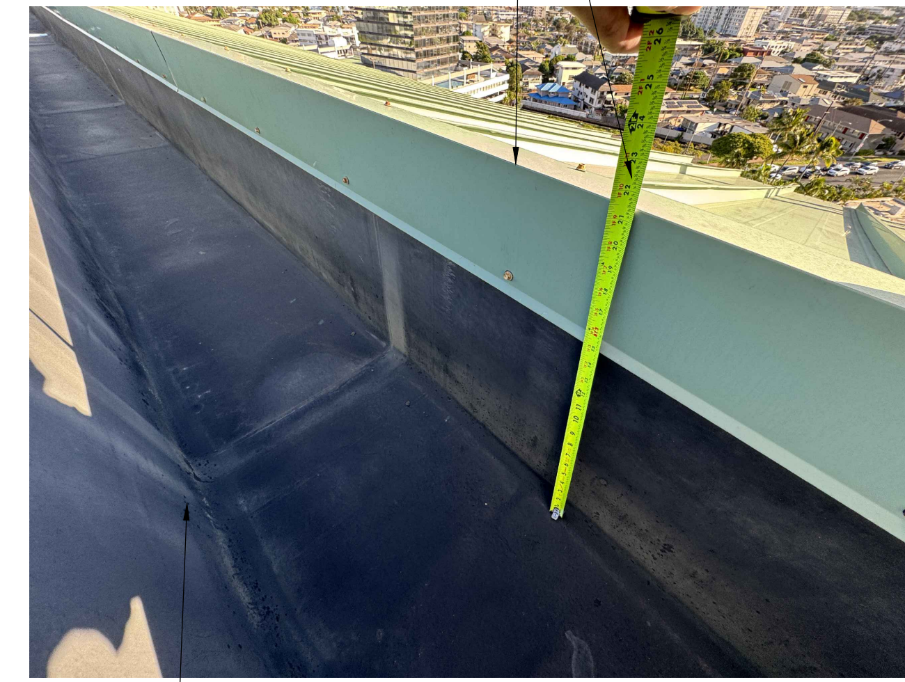
NOTE: 1. ALL (E) EXPOSED FASTENERS TO BE REMOVED AND REPLACED, REFER TO WP1.01 & WP1.02 2. LAPPED JOINT TREATMENT, SEE 6/WP9.01 EXISTING CONDITION PHOTO REFERENCE 1 N.T.S. DO NOT SCALE PHOTO REFERENCES. WP9.01
