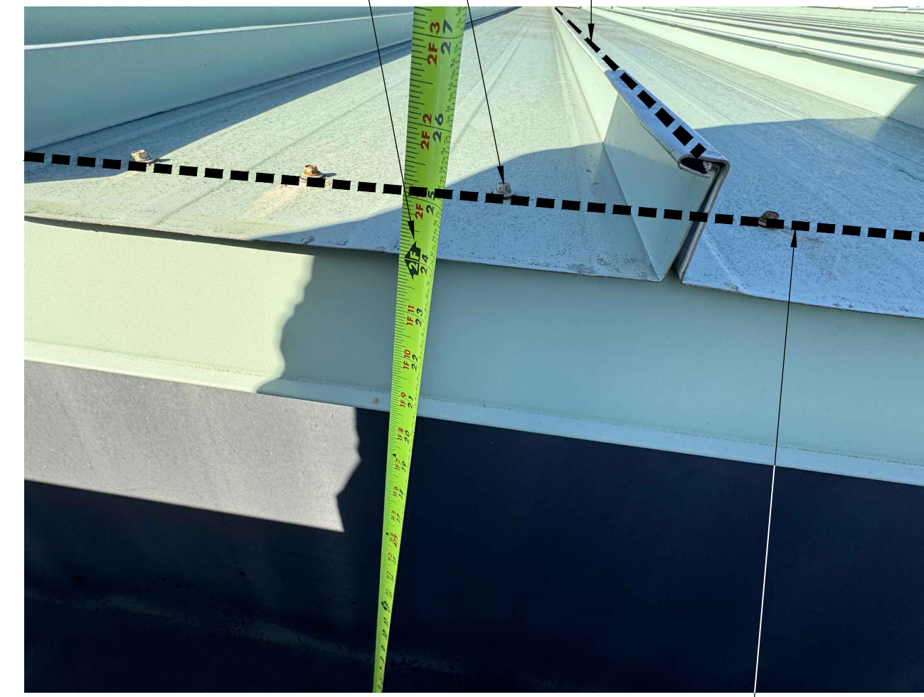
NOTE: 1. ALL (E) EXPOSED FASTENERS TO BE REMOVED AND REPLACED, REFER TO WP1.01 & WP1.02 EXISTING CONDITION PHOTO REFERENCE 7 N.T.S. DO NOT SCALE PHOTO REFERENCES. WP9.01
