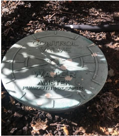
Irrigation Control Box – Typical
