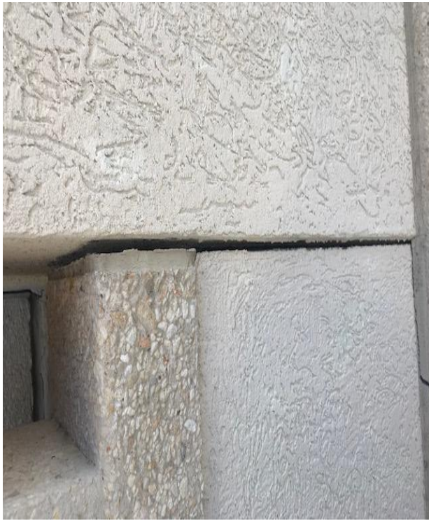
Wall Condition at EFIS
