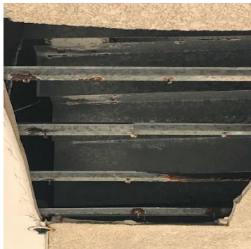
Condition Underneath Planter Boxes in Various Areas
