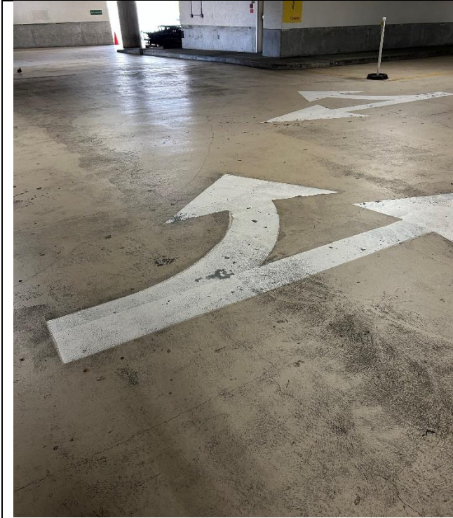
Directional arrows to be repainted following floor sealing.
