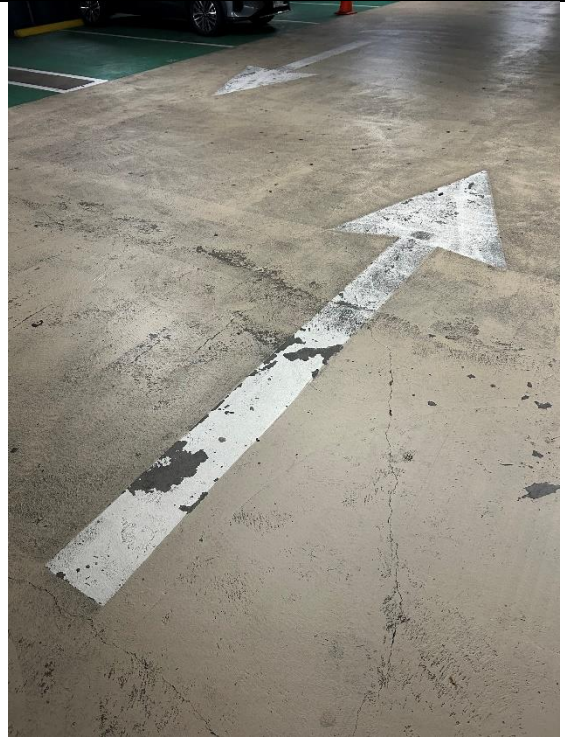
Directional arrows to be repainted following floor sealing.
