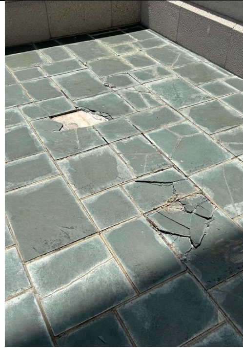
Exposed Area of 3 rd Floor Concourse
